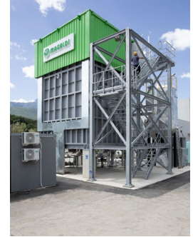
Magaldi's fluidised bed TES system (single tank)
