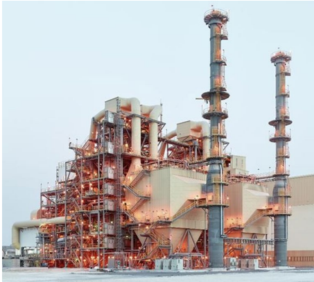
Outotec's 5th Gen CFB alumina calciner
