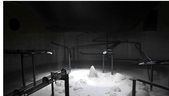
Magaldi's fluidised bed TES system (single tank)
